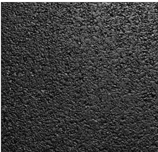
PAVING TYPE 4: BITUMEN MACADAM TO ROADWAYS, RAISED TABLES AND PARKING BAYS
