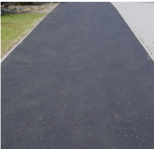
PAVING TYPE 2: BITUMEN MACADAM TO PEDESTRIAN FOOTPATHS
